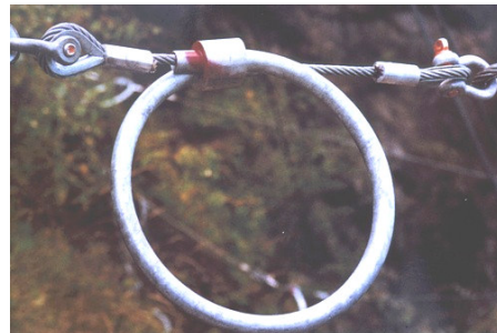
Figure 6: Details of a rockfall net system manufactured by Geobruigg of Switzerland.
