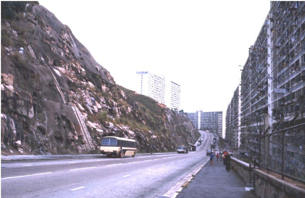
Figure 1: A view down Sau Mau Ping Road in Kowloon showing apartment blocks across the road from the steep rock slopes.
